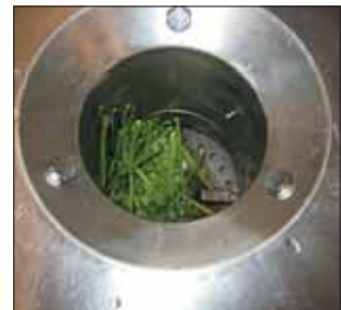
View of waste inlet with water flushing nozzles
